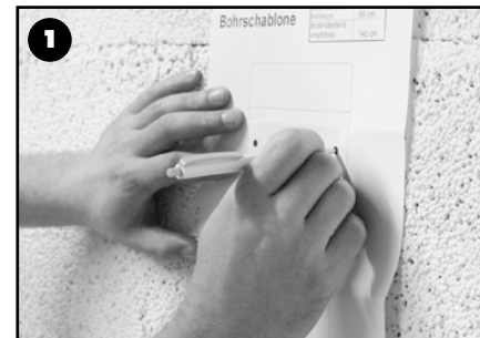
1. Place template at desired height on the wall. Mark in drill holes onto the wall.
