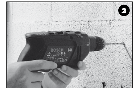
2. Drill all four holes with a 6 mm drill bit. Drill holes deep enough so that the anchors (when inserted) are flush with the wall.
